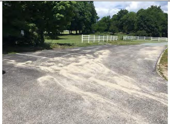
**Photo 2:** Sediment from uphill deposited on paved driveway.
