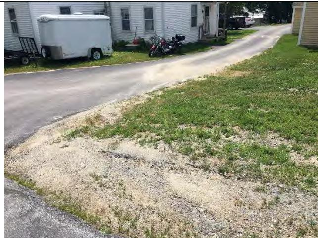
**Photo 1:** Corner of driveway being eroded and mobilizing sediment.
