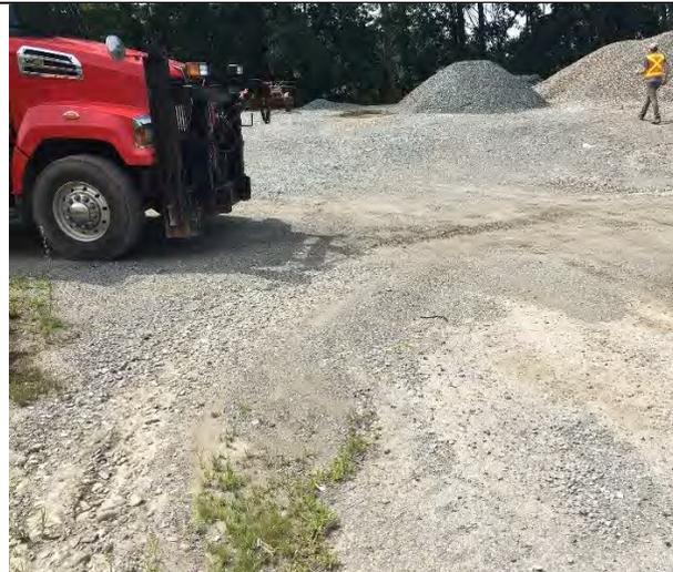
**Photo 1:** Sheet erosion in the gravel parking lot behind the garage.
