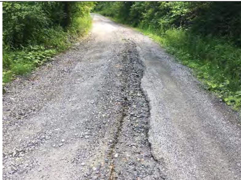
**Photo 1:** Gully erosion in center of the road from water flowing directly down ROW.
