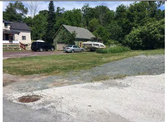
**Photo 2:** Catch basin accepting stormwater with gravel deposition around it.
