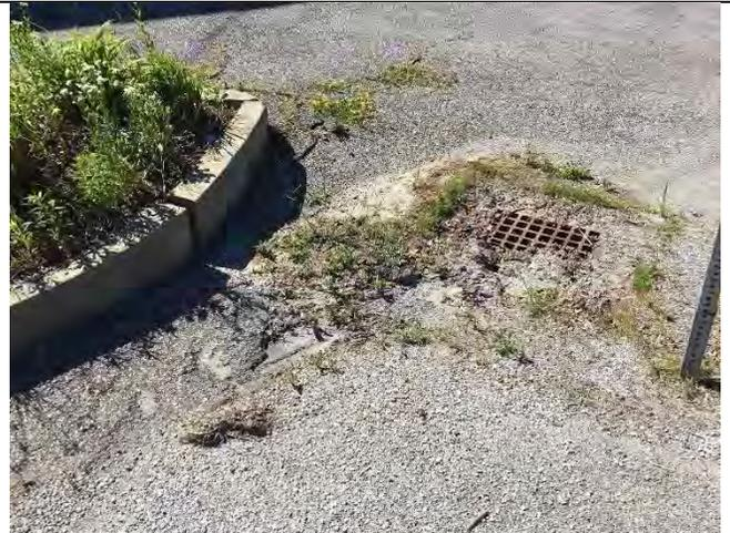
**Photo 2:** Catch basin accepting stormwater with gravel deposition beginning to clog it.
