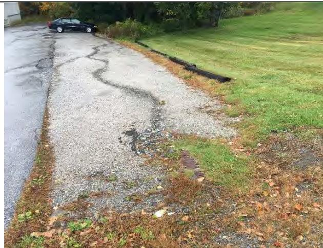
**Photo 1:** Stormwater flowing over gravel out of broken culvert
