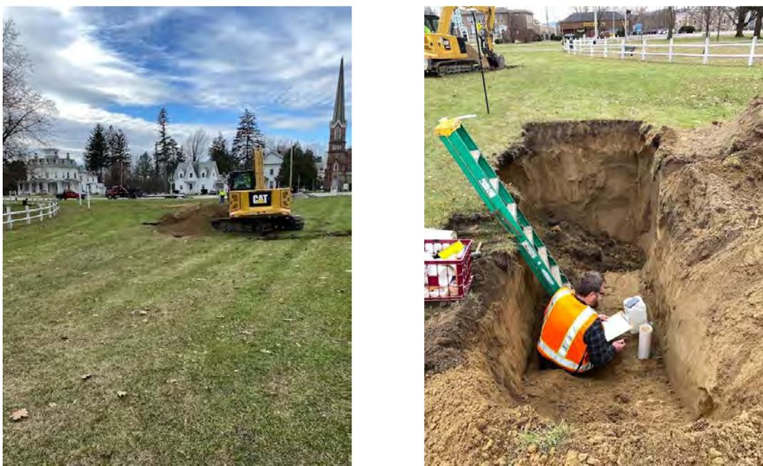
**Figure 3:** Project FHV-06 had the highest total score (31 out of 50) in the Unified Prioritization. The project is located on the north side of the Fair Haven. In fall of 2021 FEA and the Town performed test pits to verify soil suitability for a large underground infiltration practice.
