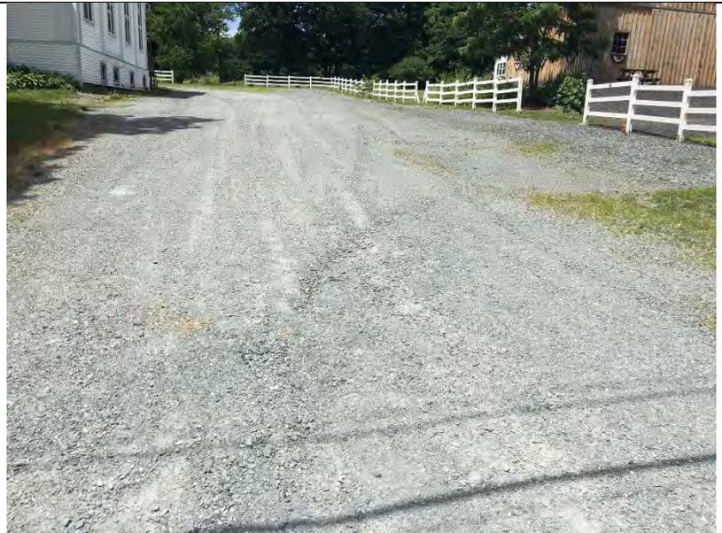
**Photo 1:** Vegetated swale accepting runoff from the church parking lot. **Photo 2:** Rill erosion in church parking lot.
