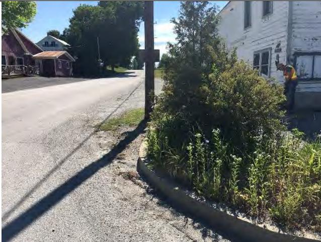
**Photo 1:** Sediment runoff along road edge.
