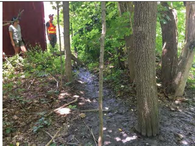
**Photo 1:** Deposited sediment from the coming from the corner of the parking lot.
