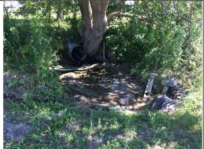
**Photo 2:** Perched culvert draining into eroded ditch before entering another culvert.
