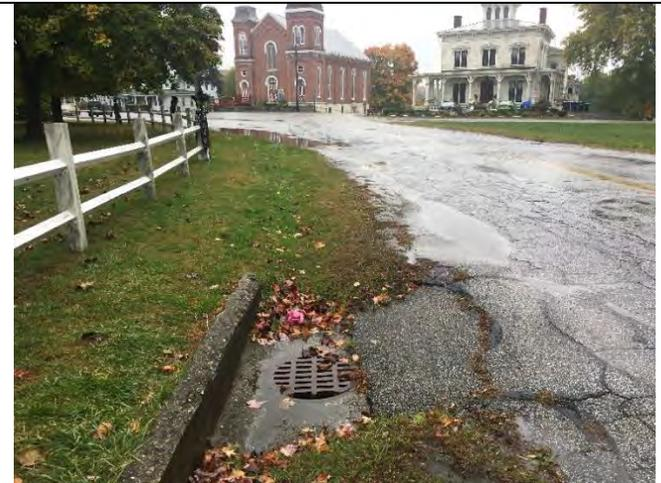
**Photo 1:** Stormwater pooling along the side of the road just up gradient from FHV-08 catch basin.
