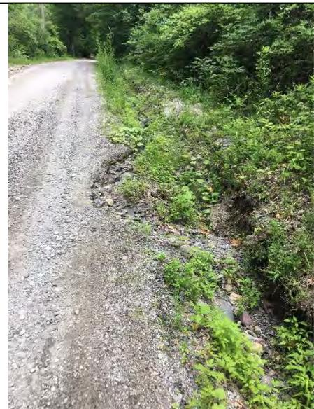
**Photo 2:** Erosion from ditch overflowing into ROW.
