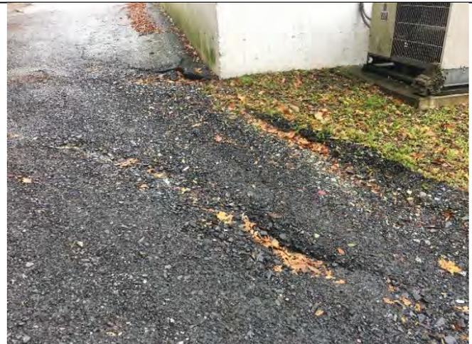
**Photo 2:** Eroding gravel in driveway just uphill of low point
