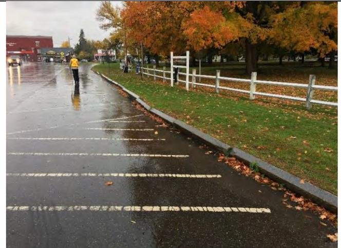
**Photo 1:** Water pooling against curb with existing catch basin far from curb and above low point
