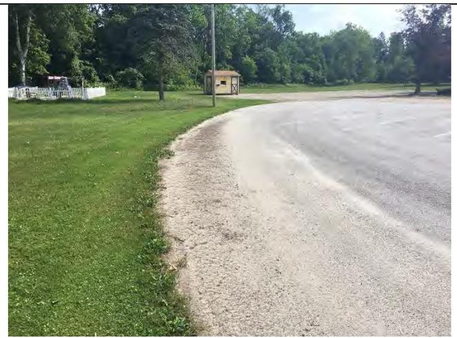
**Photo 1:** Sheet erosion in gravel portion of parking lot. **Photo 2:** Sediment deposition along the edge of the paved section of the parking lot.
