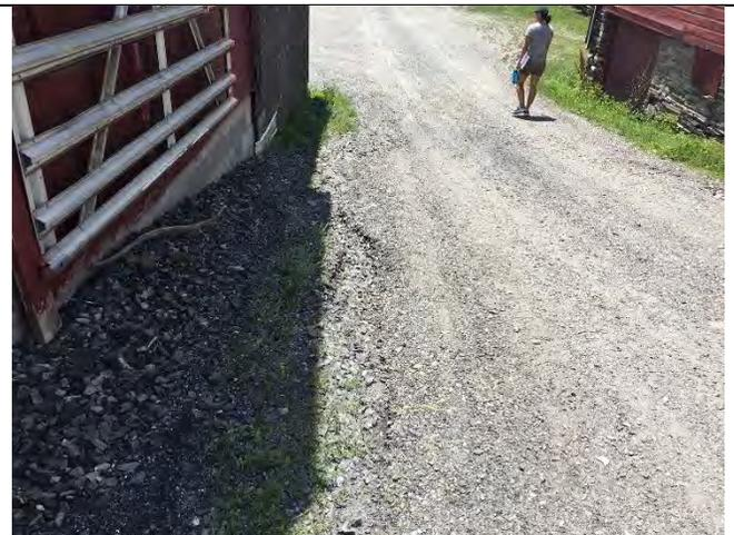
**Photo 2:** Small gully forming in steeper section of the parking lot.
