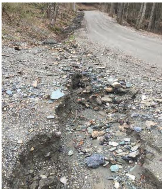
**Figure 5:** Rural roads can contribute gravel and nutrients to nearby streams. River Road in Poultney after a large spring storm (2019).
